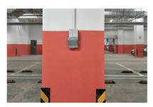
The detector is installed in each fire compartment/room. The installation location should consider the factors such as gas concentration, detection representativeness and installation convenience. The detector is connected to the controller via a network cable.
