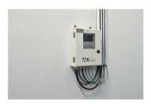
The controller has built-in multi-input and 9 relays, and can freely group the detectors to realize partition control function. At the same time, the controller built-in alarm value setting, delay start and other optional linkage needs.
